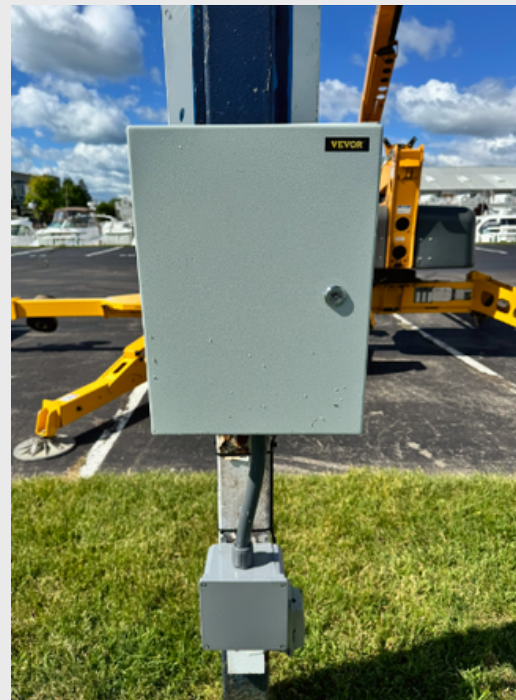
New NEMA mounted on site to upgrade the harbor's electrical and power systems
